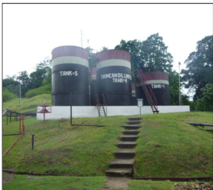
Figure 1: Trinidad Oil Tank Battery
