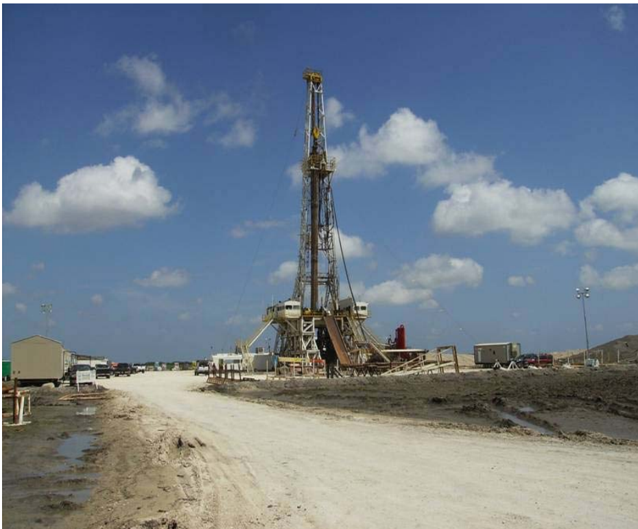
Figure 1: Unit Texas Rig #35 on Smith #1 well
