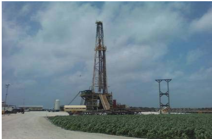
Figure 5: Precision #37 rig drilling ahead on Russell Bevly #1 Well
